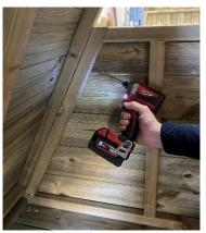
5. After securing the back panel and after some slight adjustment secure the peak of the product using 4 x 80mm screws
